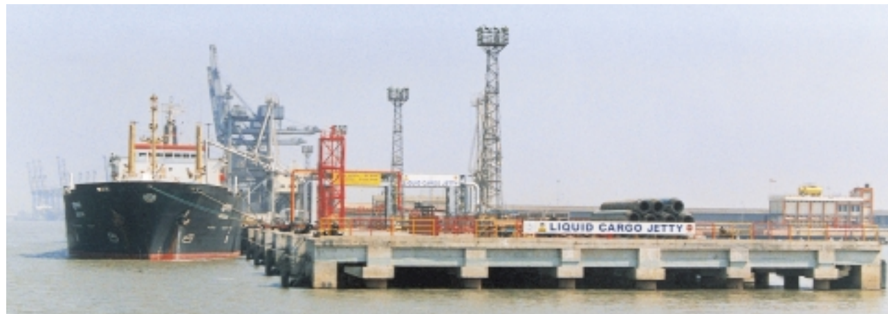
Liquid Cargo Jetty at JNPT, Maharashtra.
