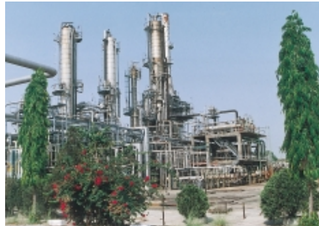
A view of Xylene Plant at BRPL Refinery.
