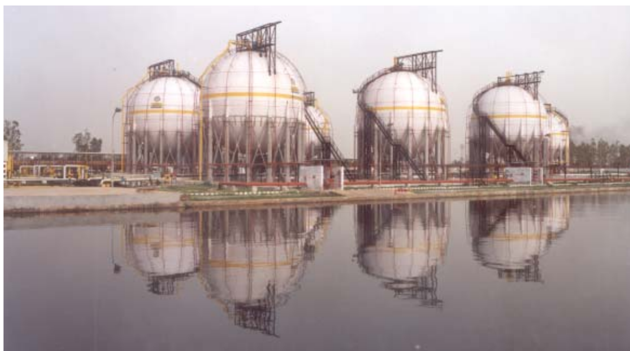
BPCL's LPG Tanks
