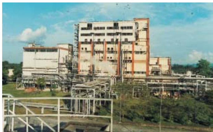
PSF Plant of BRPL
