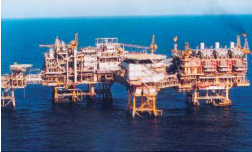
ONGC's Offshore Platform in Mumbai High
