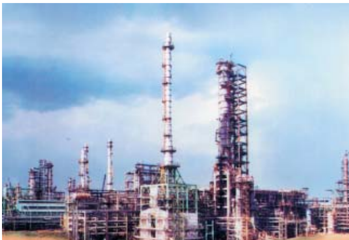
A view of CPCL's Rs. 2360 crore 3MMTPA capacity expansion and modernization project at Manali
