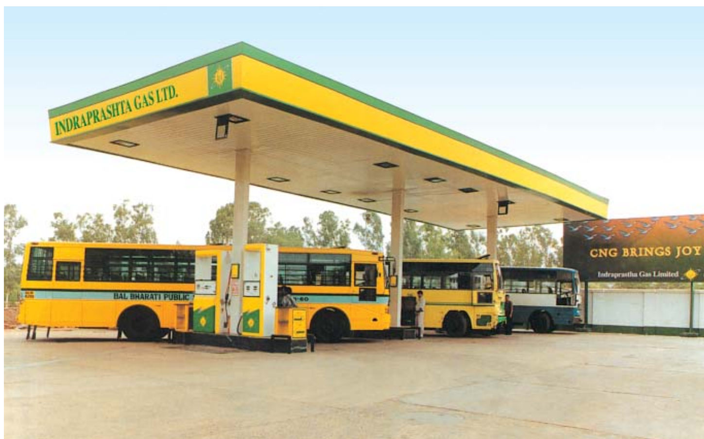
A CNG filling station : a step towards pollution control
