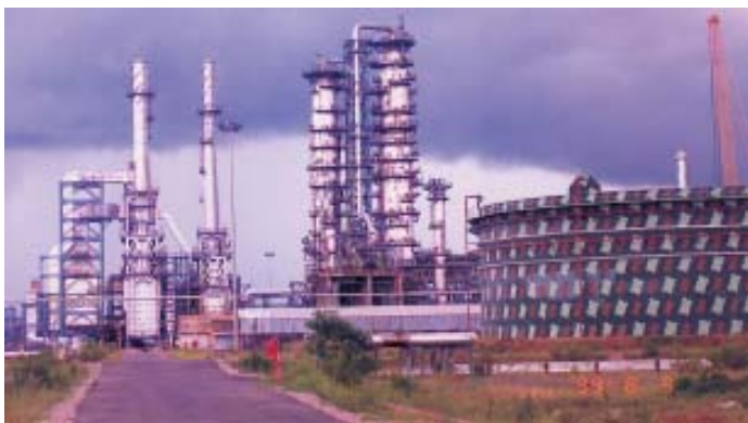
A view of NRL's Refinery
