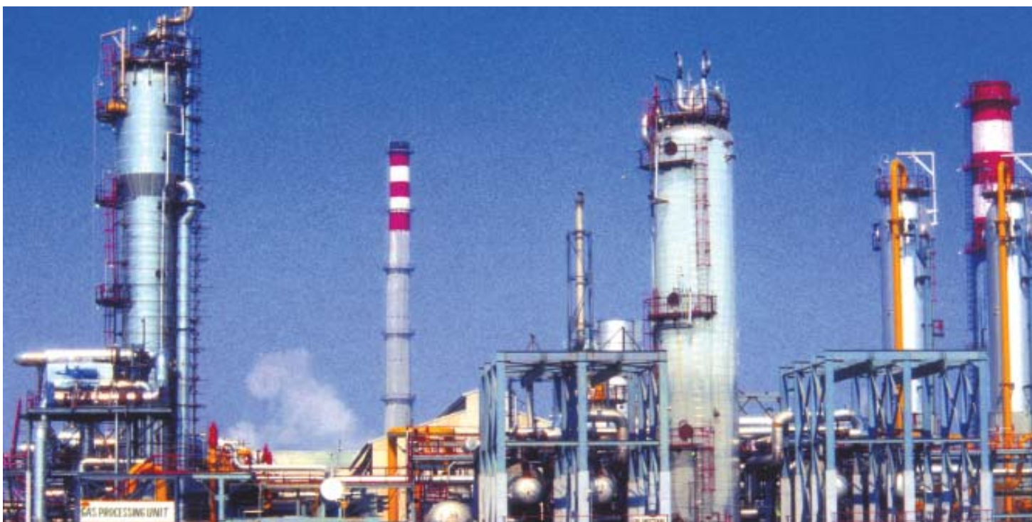
Gas processing unit of GAIL
