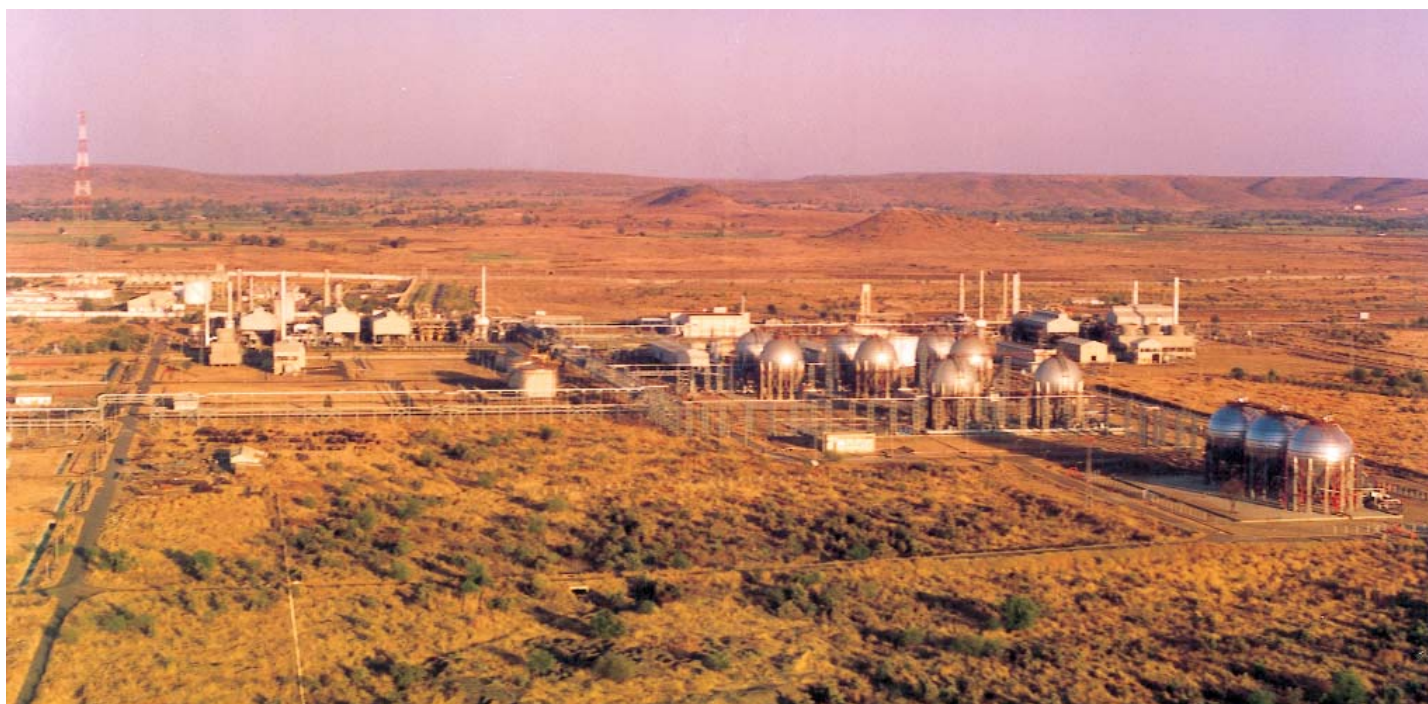
Aerial view of Horton Sphere at LPG recovery unit - Vijaipur (GAIL)
