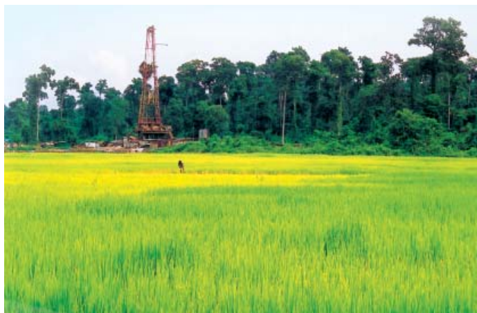
Drilling Operations in Assam – Oil India Ltd., like all other oil PSUs ensures Environmental Protection while carrying out its operations
