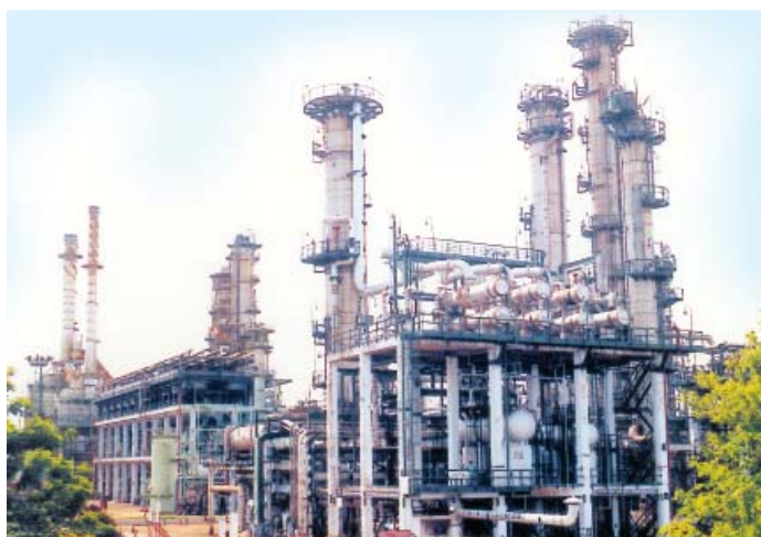
A view of the Kochi Refineries Ltd.
