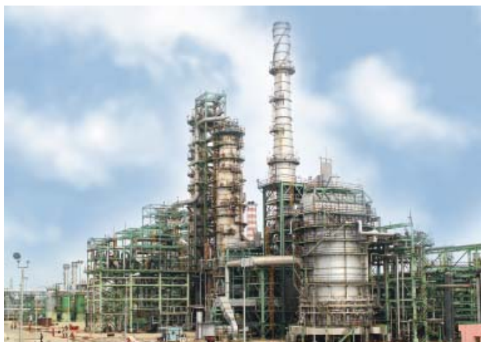
A view of CPCL's Crude Unit at Refinery III Complex, Manali
