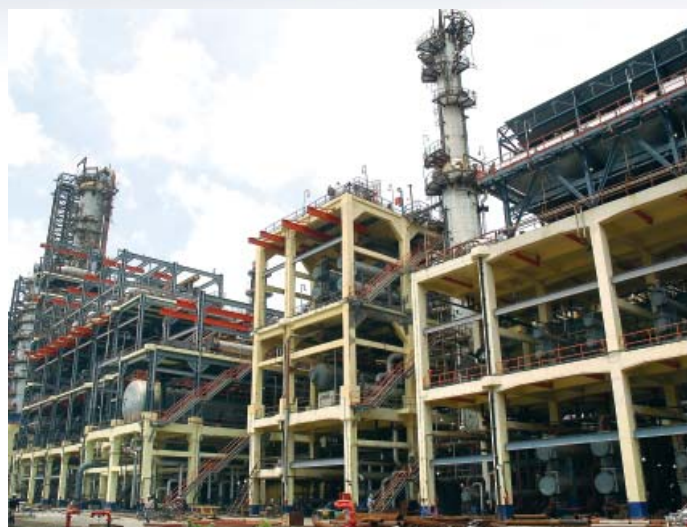
A view of BPCL's Refinery Modernization Project
