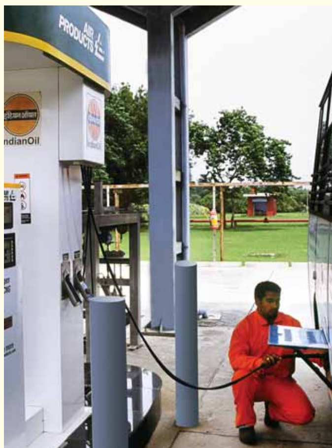
India's first experimental Hydrogen-CNG dispensing station set up at Indian Oil's R&D Centre for trials on select vehicles on way to commercialisation of Hydrogen as an alternative automotive fuel.
