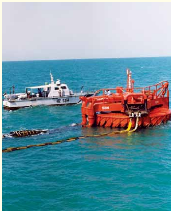
Single Buoy Mooring at Vadinar in the Gulf of Kutch for receipt of imported crude oil through Very Large Crude Carriers.
