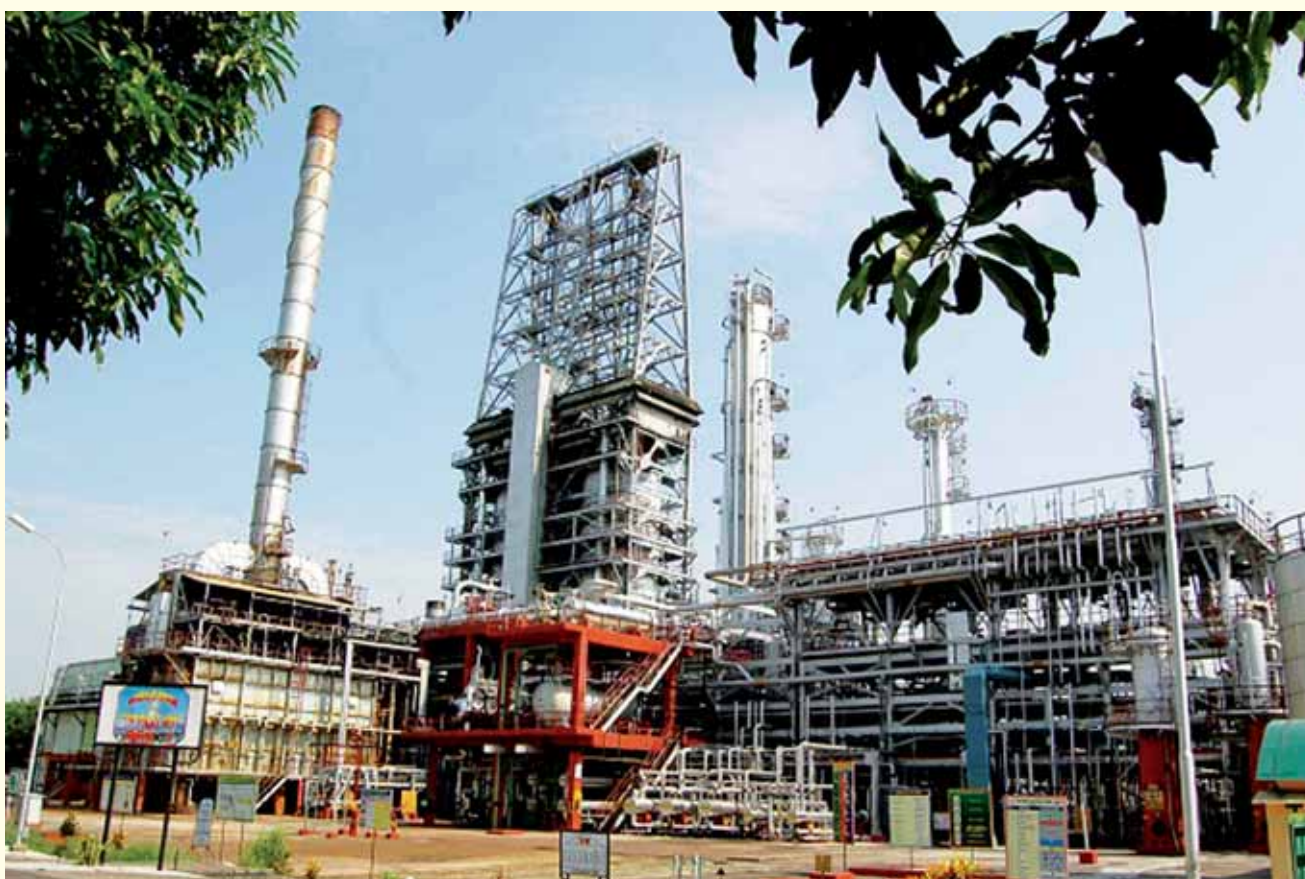
A view of the Delayed Coking Unit (DCU)-I of BRPL after implementation of TPM.
