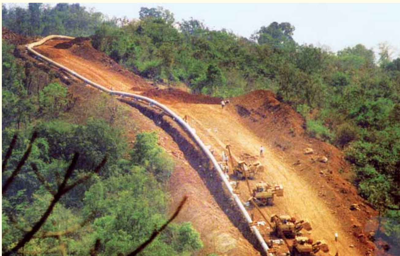
Laying of GAIL- Dahej-Uran Pipeline for Natural Gas transmission
