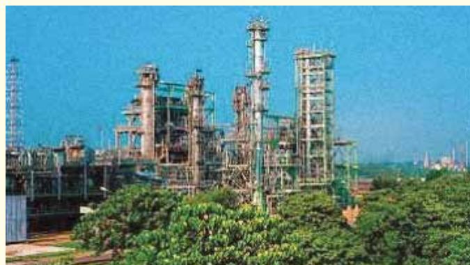
A view of BPCL's Kochi Refinery
