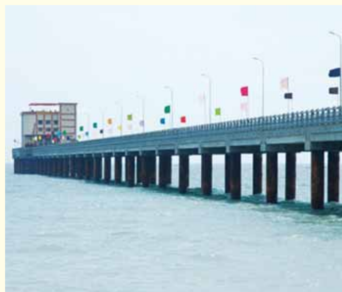
A view of CPCL's 5.8 MGD Desalination Plant at Kattupalli near Ennore
