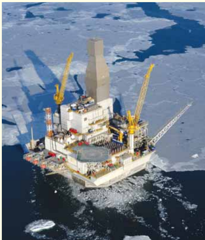
An installation at Sakhalin in Russia, where ONGC Videsh is operating to bring in equity oil for India
