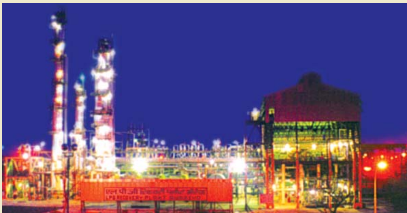
Night View of LPG Recovery Unit at Pata, Distt Auraiya, U.P.
