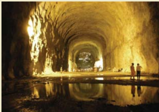
Crude oil storage cavern at Visakhapatnam
