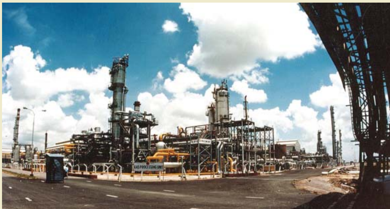
Gas Processing Unit of GAIL at Pata, District Auraiya, U.P.
