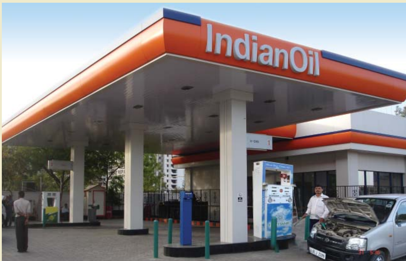
H-CNG Dispensing station at Dwarka, New Delhi
