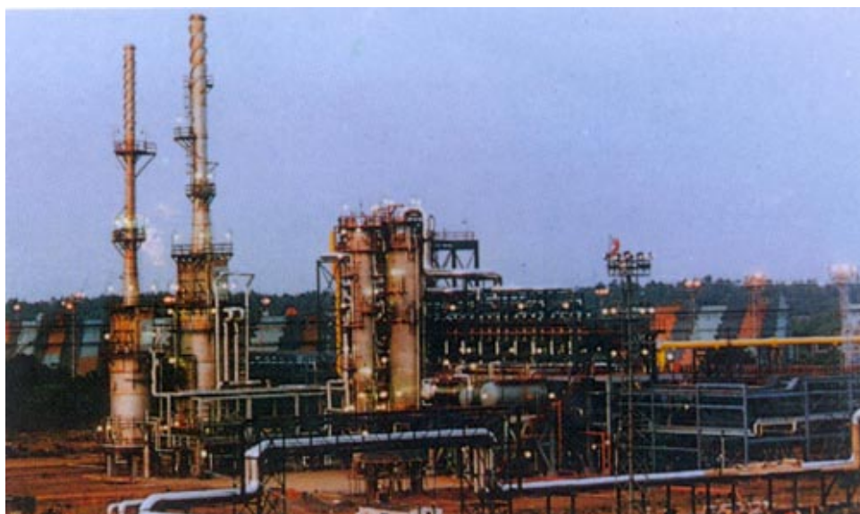
Hazira Processing Complex at Hazira of ONGC
