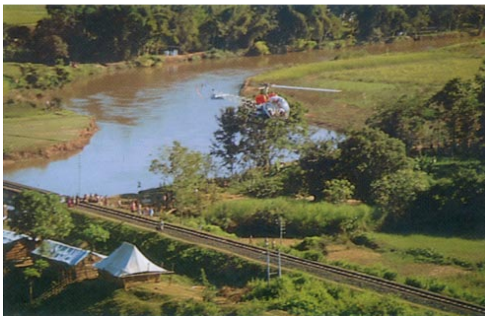
Inspection of OIL's Crude Oil Pipeline at a river crossing in Lower Assam
